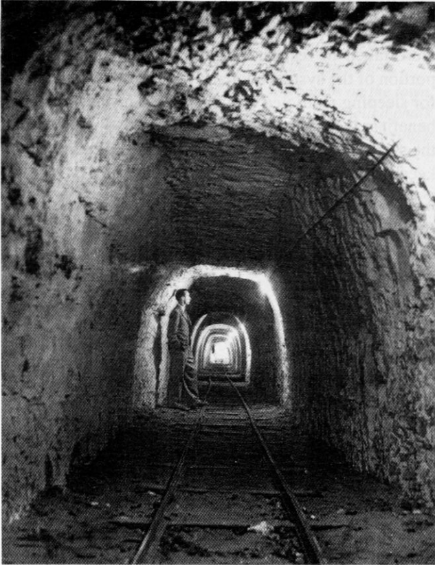
A temporary contractor's railway was laid during construction of the tunnels
